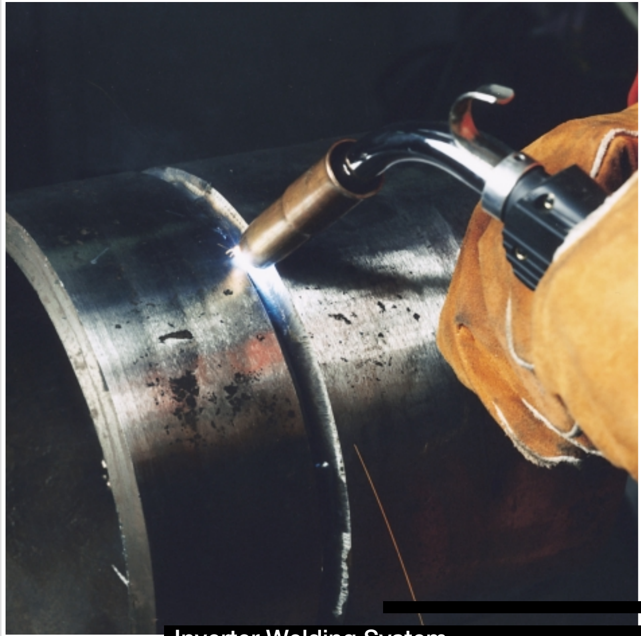
Inverter Welding System
